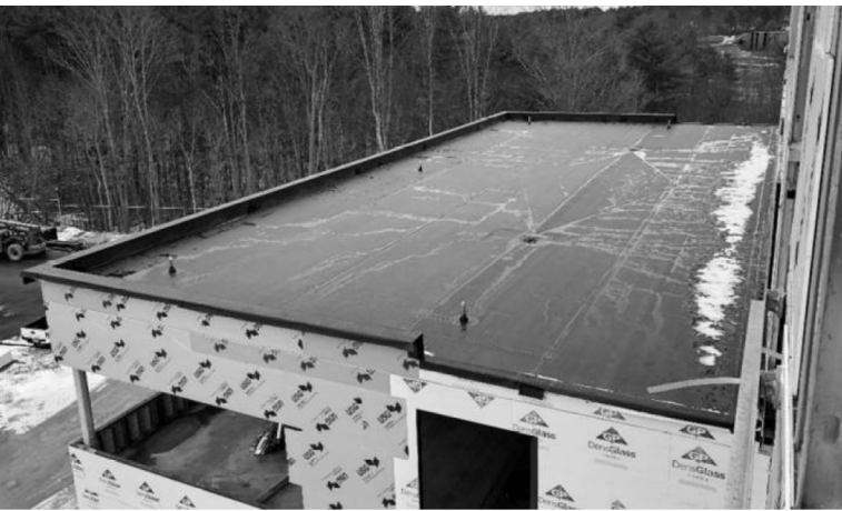
View of roof at Gym
