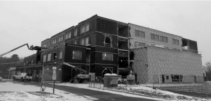
View of South-West Elevation
