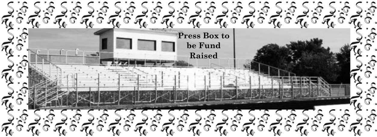
1000 seat bleachers to be constructed in time for the Class of 2021 June 11, 2021 graduation and to be dedicated to both the Class of 2020 and the Class of 2021!
