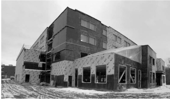
View of South-East Elevation
