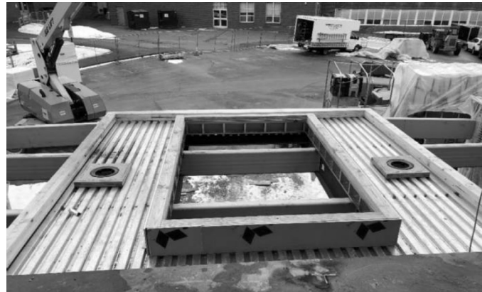
View of main entry roof canopy
