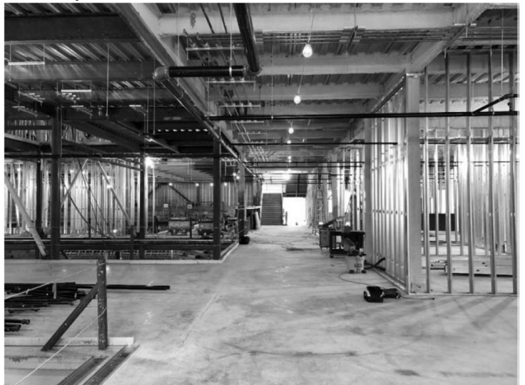
View at Second Floor looking towards Stair D
