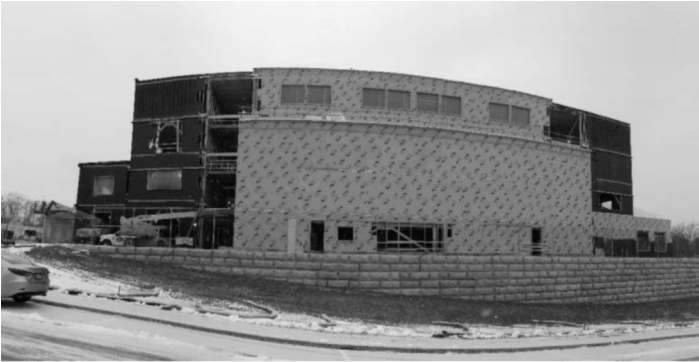
View of South Elevation
