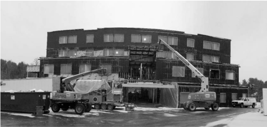
View of West Elevation
